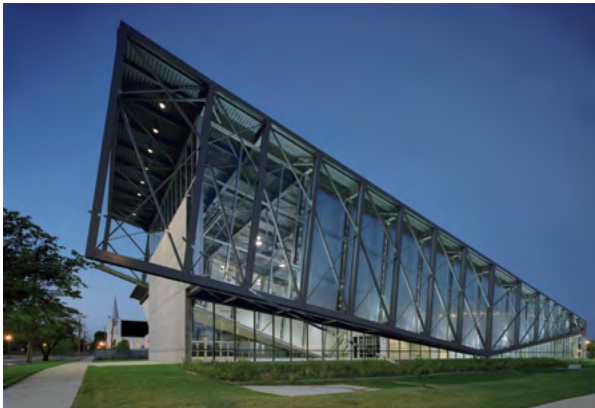
Jim Boyd Bridges Center Bridges USA, Memphis, TN Completed 2004
