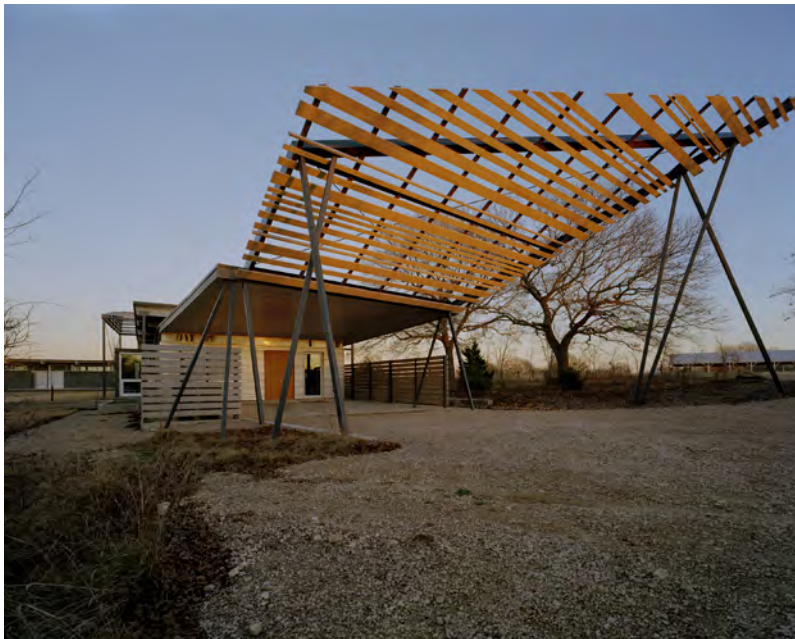
Texas Twister Rey Rosa Ranch, Dallas, TX Completed 2002 Photo: Timothy Hursley
