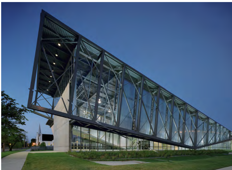
Jim Boyd Bridges Center Bridges USA, Memphis, TN Completed 2004
